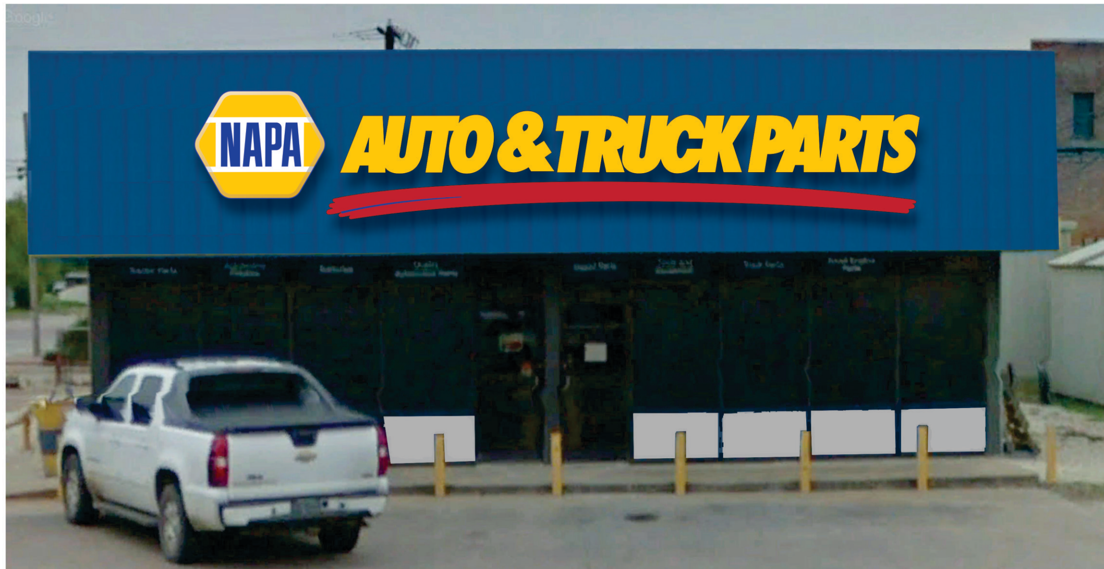
One (1) NEW LED ILLUMINATED Logo, Letterset & Swoosh Direct Mounted on Building Fascia
